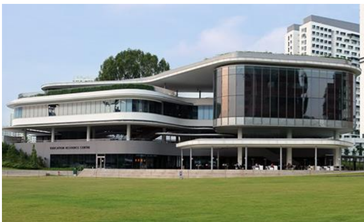
Education Resource Centre Building
